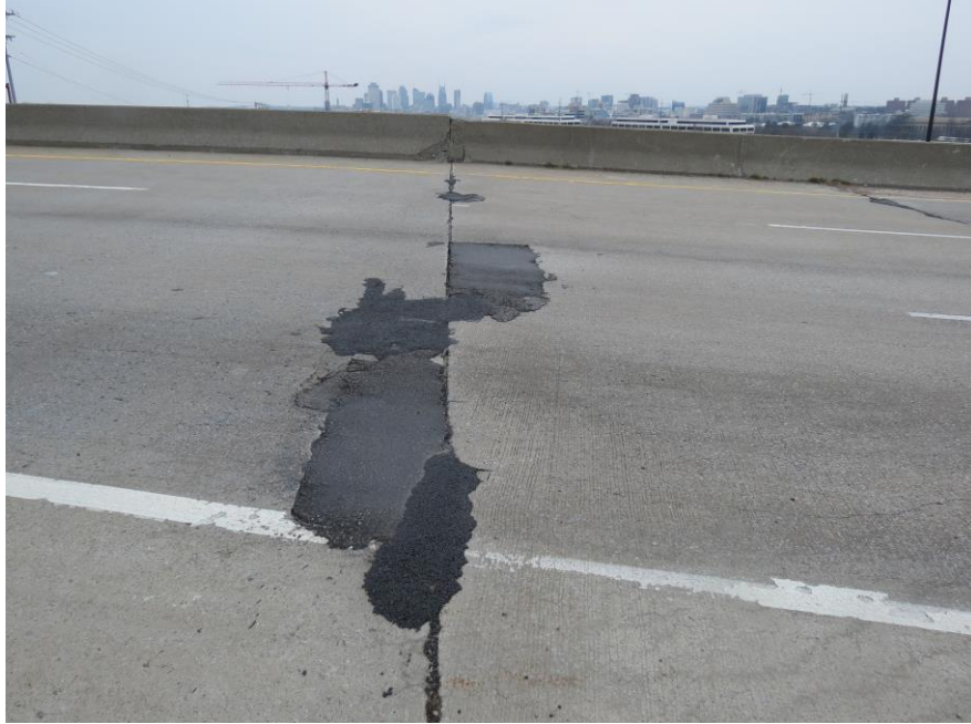
APPR. "B" END JOINT W/ PATCHES
