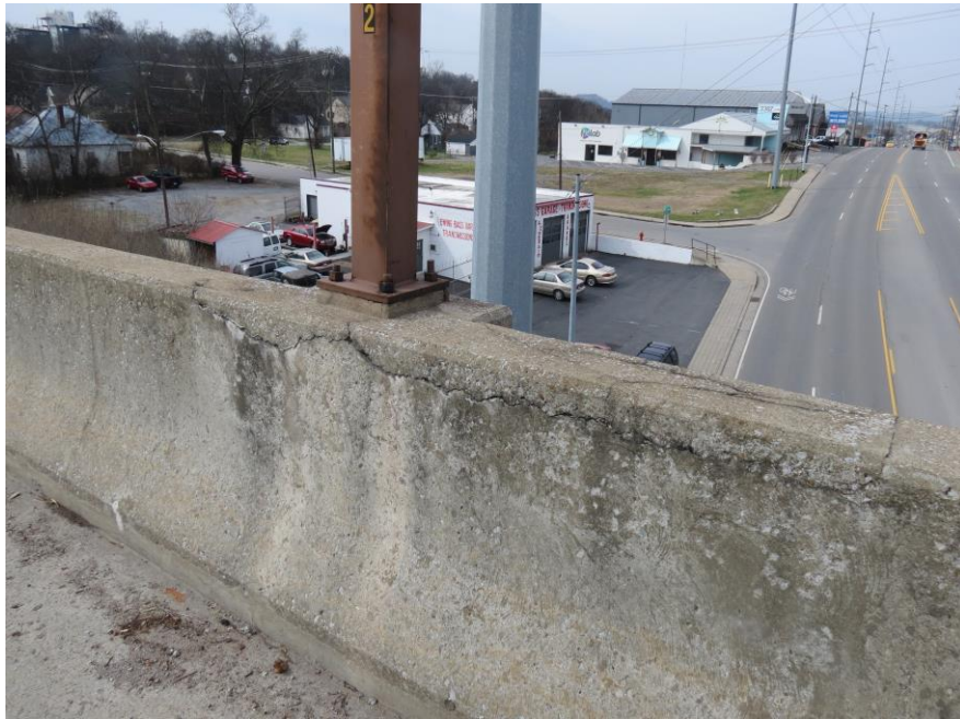
PARAPET RT. W/ I.P.B.O UNDER POLE ID # HM02
