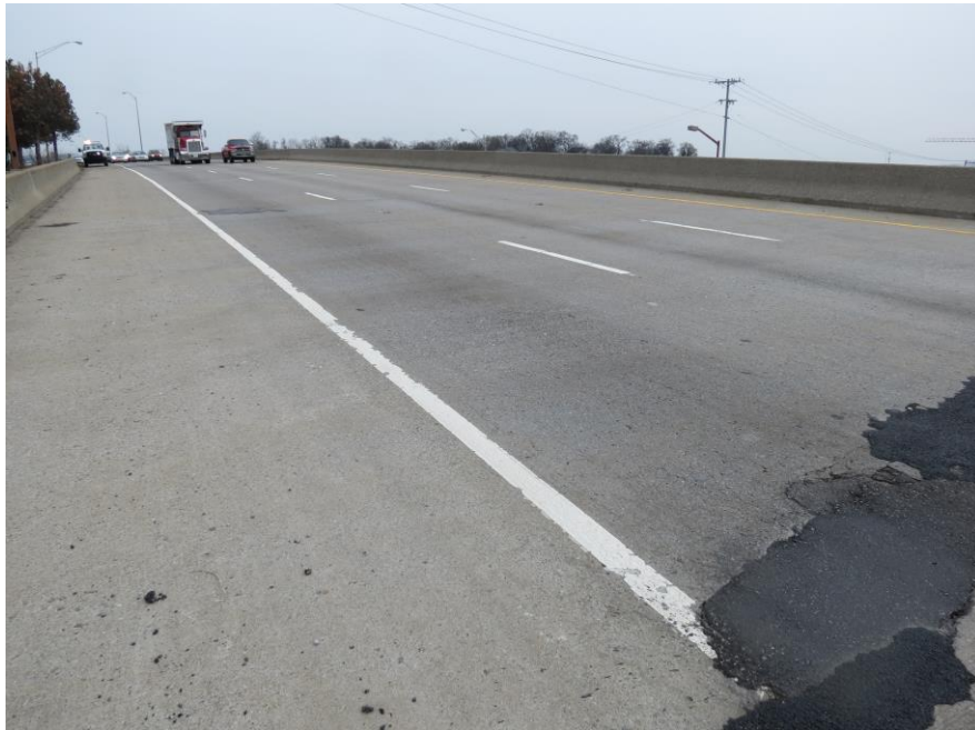
VIEW ACROSS TOP OF WEARING SURFACE
